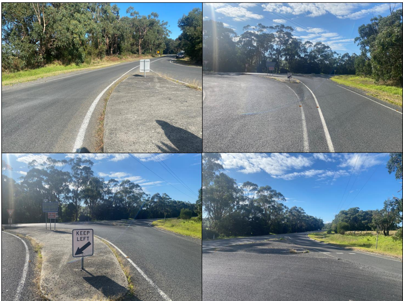
Figure 1-11 Site No. 3 – Inspection Images
