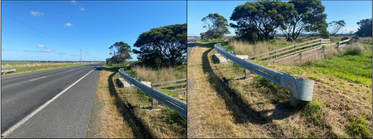
Figure 1-26 Site No. 9 – Inspection Images
