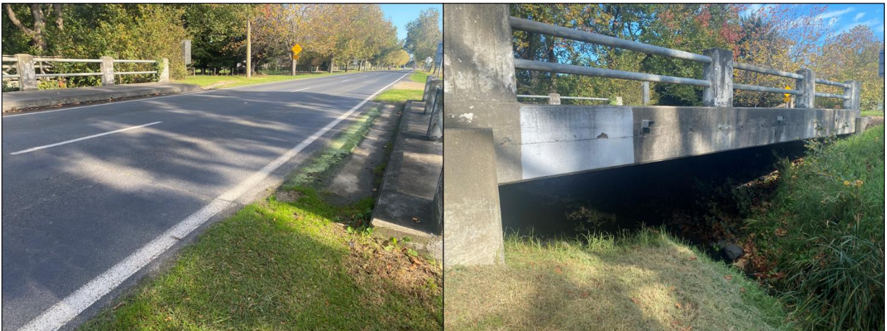
Figure 1-13 Site No. 4 – Inspection Images
