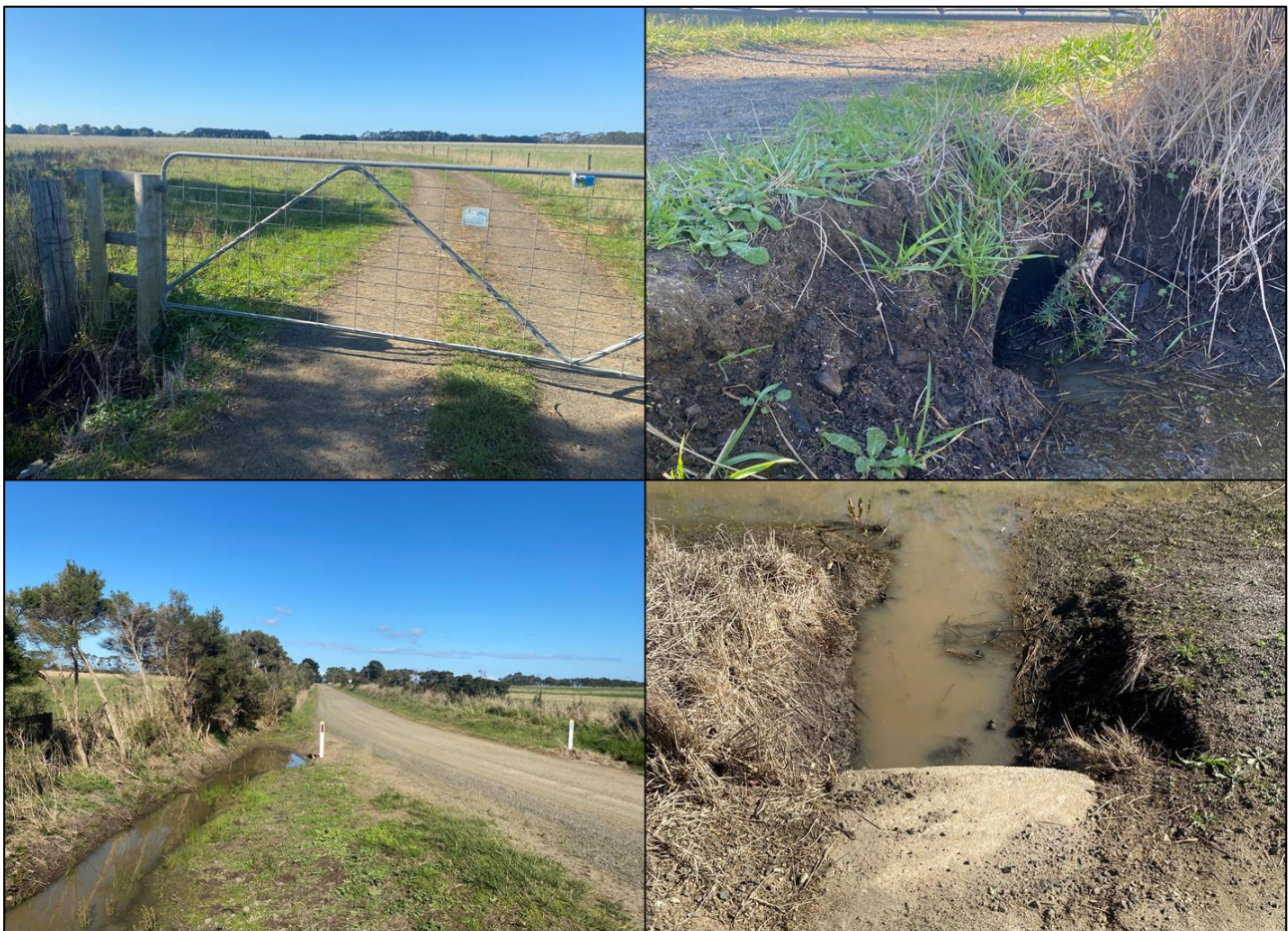
Figure 1-32 Site No. 12 – Inspection Images
