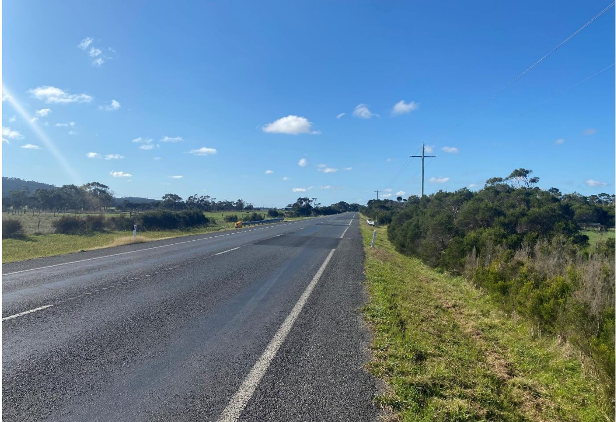
Figure 2-2 South Gippsland Highway looking north-east near Site Access 1
