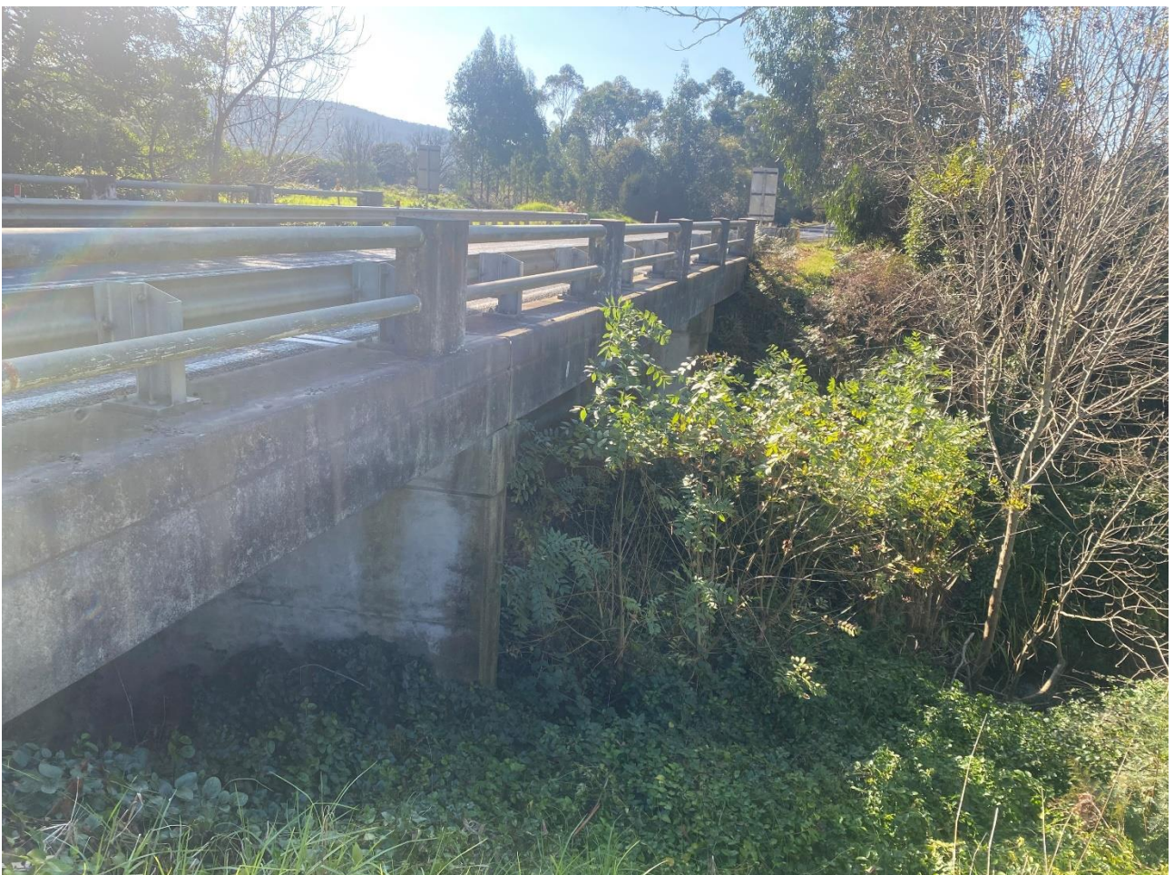
Figure 1-15 Site No. 5 – Inspection Images
