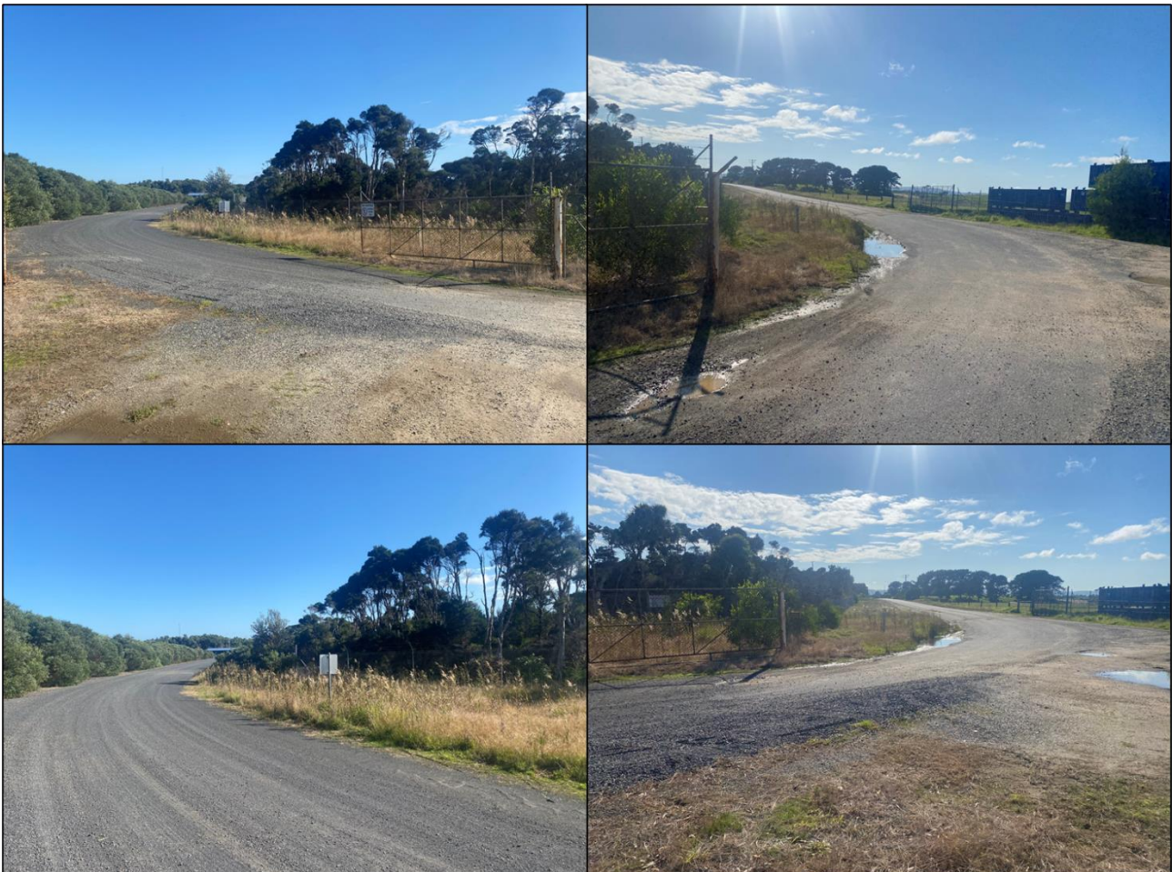
Figure 1-7 Site No. 1 – Inspection Images
